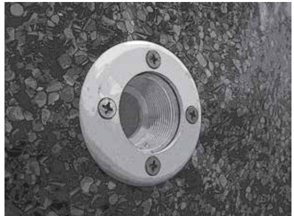
Return faceplate installed.
