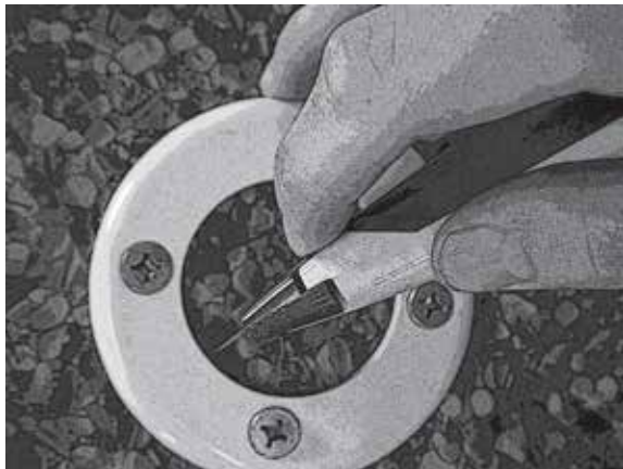
Trim liner from return opening.
